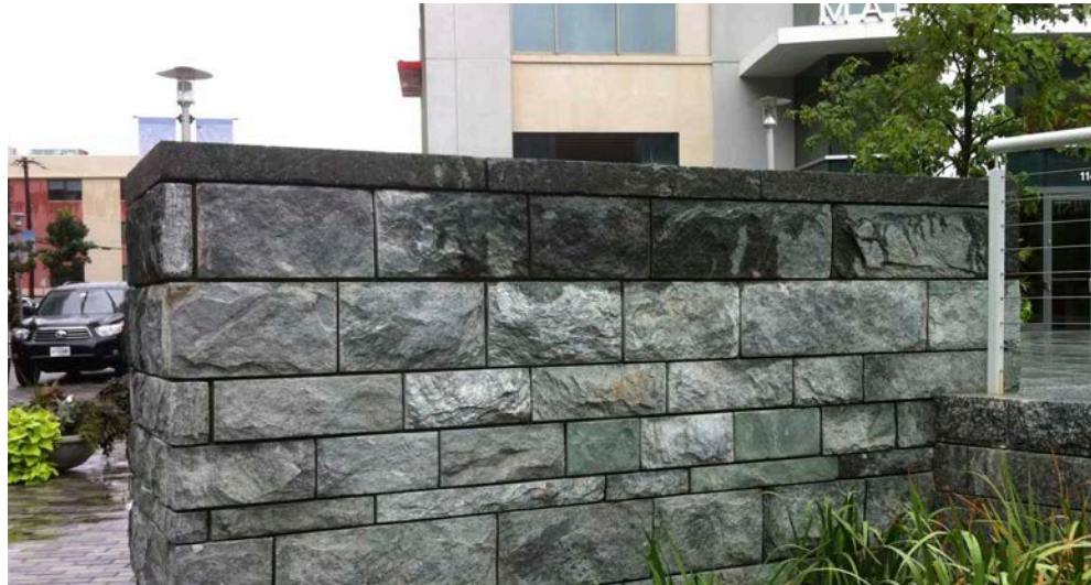
Carderock Retaining Wall
